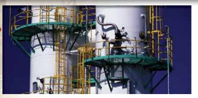
Fuel gas valves to furnaces in a petrochemical plant ethylene cracking unit. Hydrocarbon feedstock is thermally cracked at high temperatures. Complexity of cracking process dictates tight control for optimal yield.
